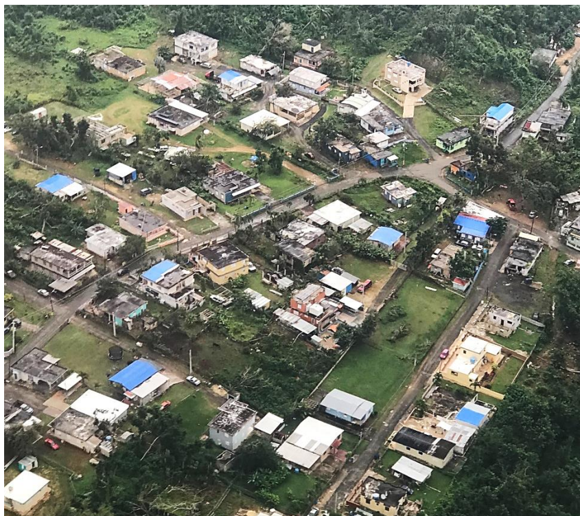
Figure 1: Blue Roofs Covering Homes in Arecibo, Puerto Rico (Feb. 21, 2018)
