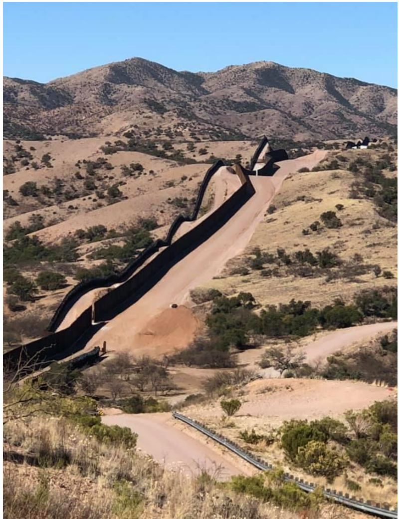
Figure 3. Incomplete Border Wall in Arizona
