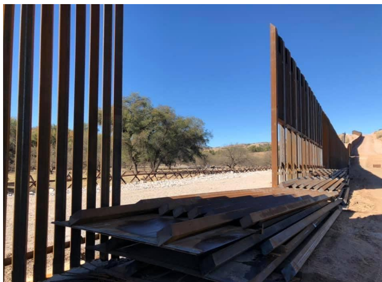
Figure 1. Incomplete Border Wall in Arizona
